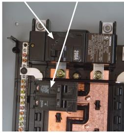
To activate standby power the utility main breaker must be in the "OFF" position to prevent dangerous feedback between the power sources.
